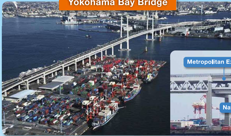
Yokohama Bay Bridge
